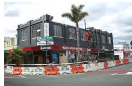
A damaged building after the Gisborne earthquake.
