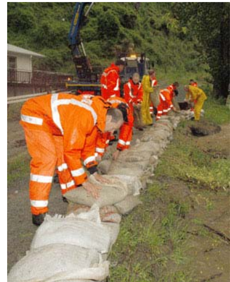
Members of NZRT2 help sandbag during a recent flood event.
